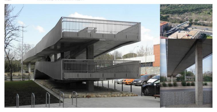
The so-called "Puente de los Franceses" Footbridge crosses the M-30 Ring-Road, connecting the Plaza de Santa Pola with the Casa de Campo. The main section is composed of a steel girder which is embedded into four columns distributed in a two-two set-up. The separation between columns horizontally is 34.0m and between the two-two set-up 3.0m. The central girder has a cantilevered area at the ends which connects with the footbridge's access ramps.
